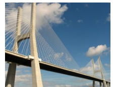
Vasco da Gama Bridge (PT)
