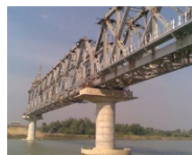
Bhagirathi Rail Bridge (IN)
