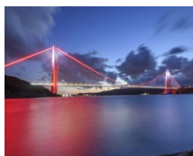
3 rd Bosphorus Bridge (TR)
