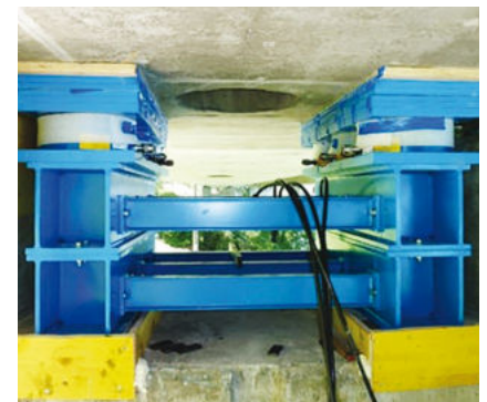
Lifting and lateral adjustment works
