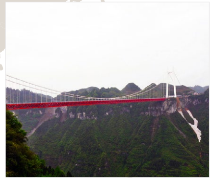
Aizhai Bridge | China
