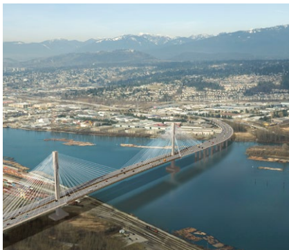
Port Mann Bridge | Canada
