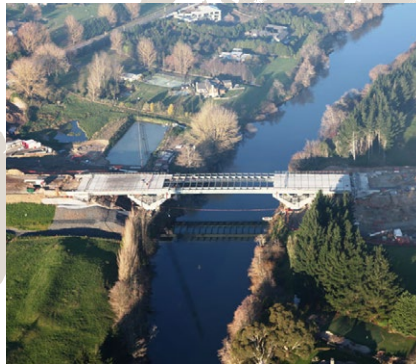
Waikato River Bridge | New Zealand
