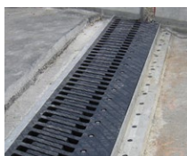
Sliding finger joint
