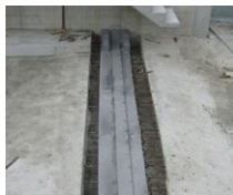
Joint prior to concreting
