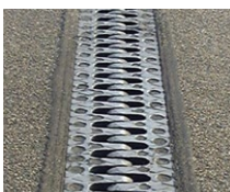
Cantilever finger joints
