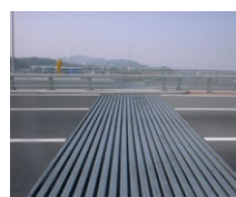
Modular expansion joints
